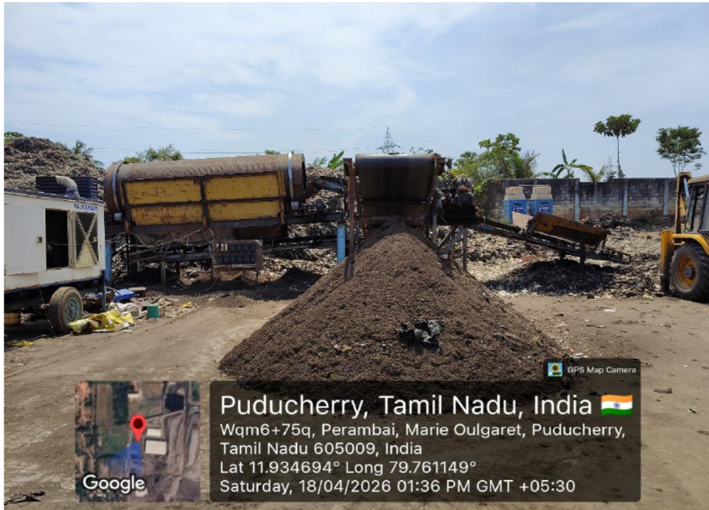
Figure 3: Solid Waste Processing Facility Established on Reclaimed Area
