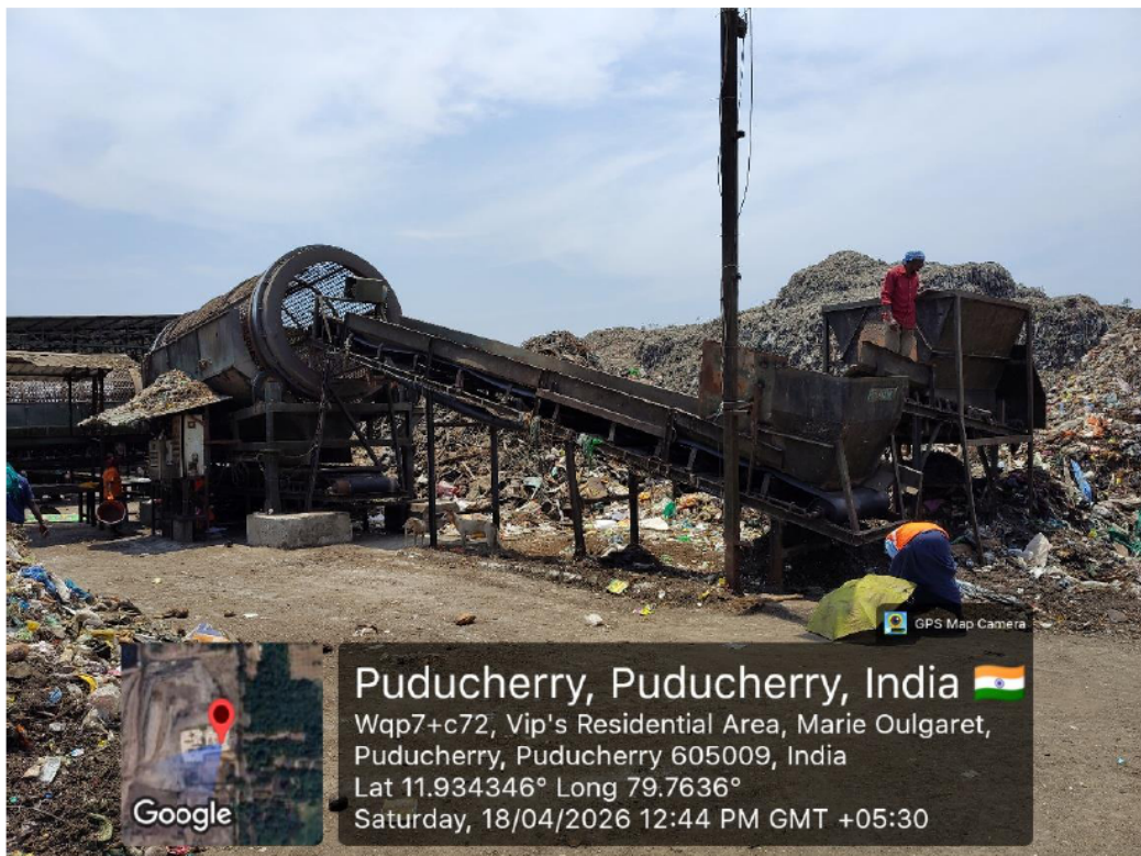
Figure 2: Solid Waste Processing Facility Established on Reclaimed Area
